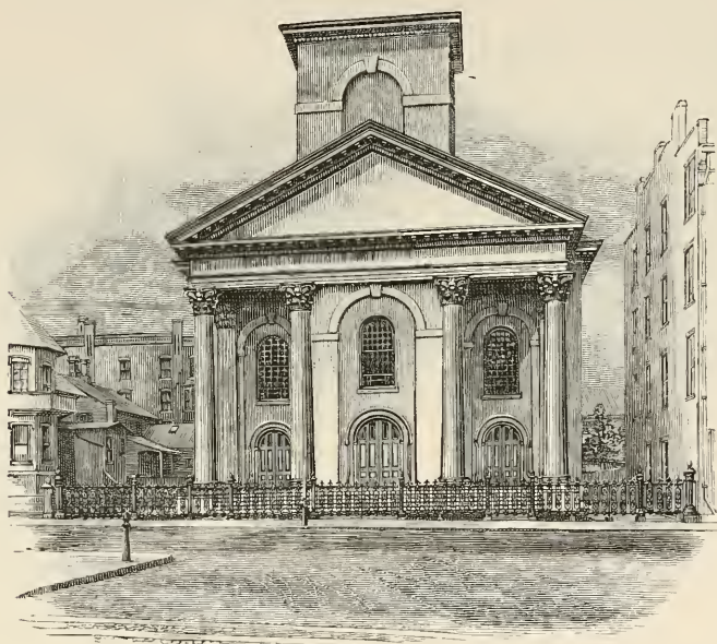
THE SECOND CONGREGATIONAL CHURCH, 1857-1894.
